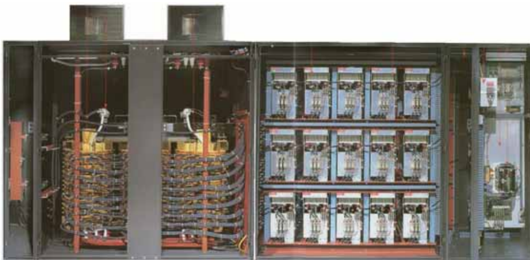
Figure 27. Example GE Innovation Series® Type H Multilevel MV Voltage Source PWM Inverter Using 5 LV IGBT Drives in Series Per Phase, Integral Power Transformer (Paice Design)
