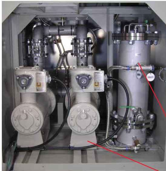
Water conditioning system behind Gate Drive Panel
