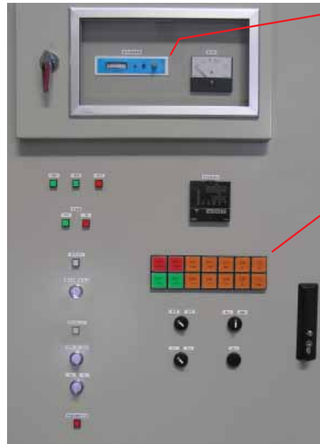
Interface and Water Cooling Panel
